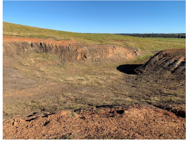
Plate 7: Example of earthworks for dam construction facing south
